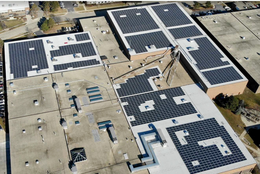
Solar array at Fellowes global headquarters, Itasca, Illinois, USA.
